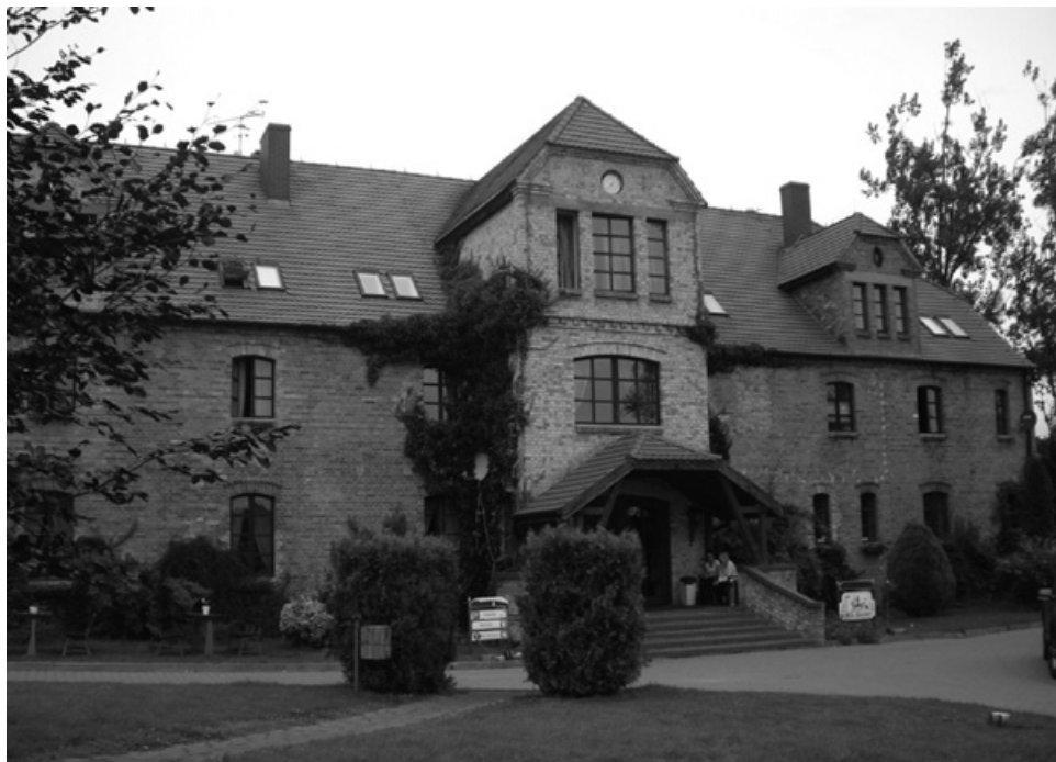
Villa Toscana. Nowe Gorzycko nr Międzychód (Western Poland). An old farm building remodeled into a hotel and restaurant. Photo W. Bryl-Roman.
